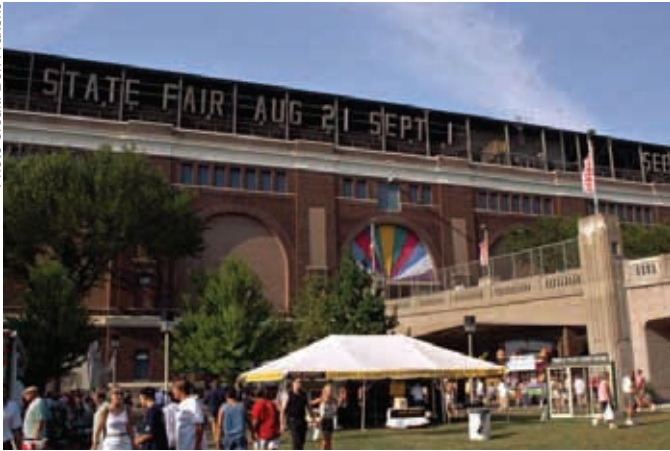
Grandstand lights and cooling units were powered by 600 kW of Rental Power from Cummins Power Generation.
