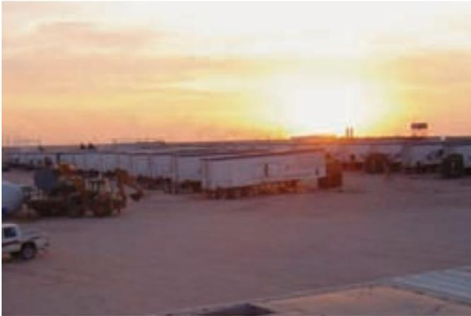
Seventy-six Rental Power units from Cummins Power Generation produce 65 MW of continuous power for pumping water to the city of Riyadh.
