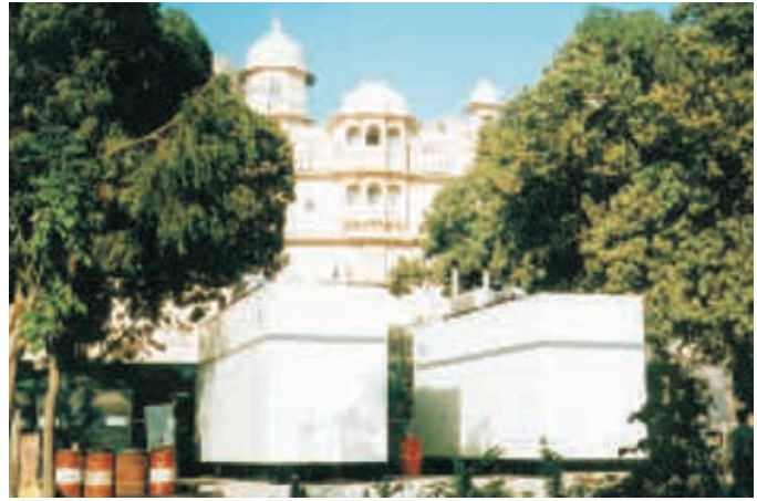
Both 750kVA generator sets were installed within the City Palace Estates.
