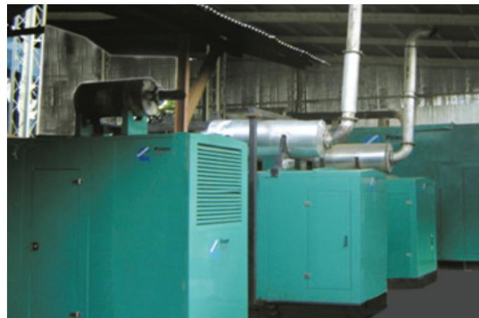
Generator sets with outputs of 250, 500 and 750 kVA were combined into complete power systems at two different sites to provide power for the shopping and residential areas of Nirmal Lifestyles.
