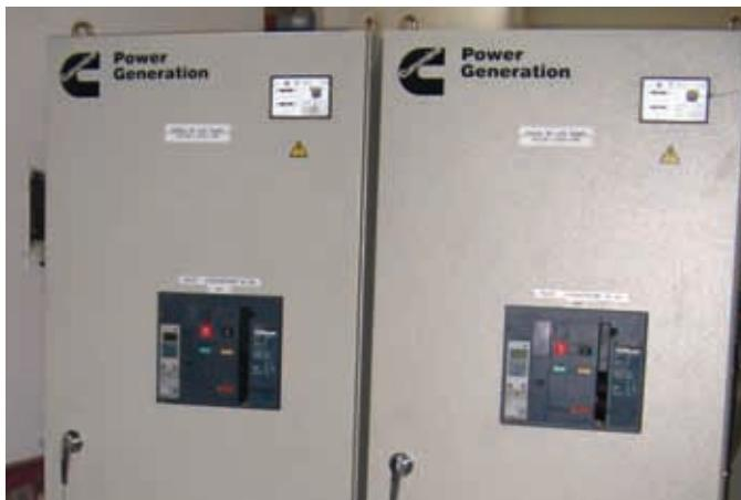
These automatic transfer switches from Cummins Power Generation monitor utility power and connect the generator to the facility's loads when there is an outage.
