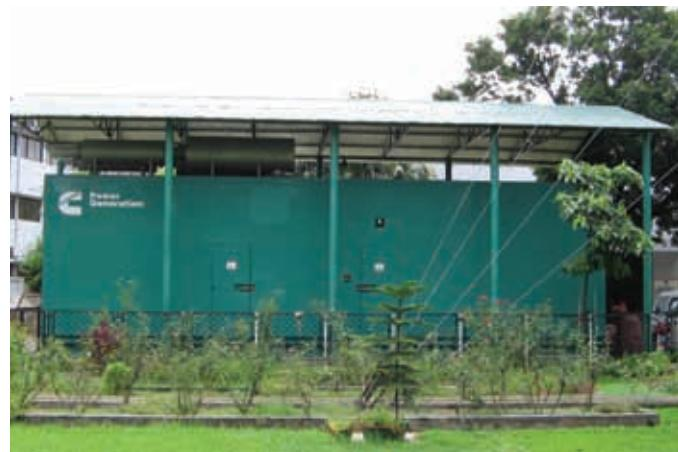
Enclosed in a sound-attenuated and weather-protected enclosure, the 2250 kVA generator from Cummins Power Generation provides the newly expanded ICDDR,B facility with mission-critical power.
