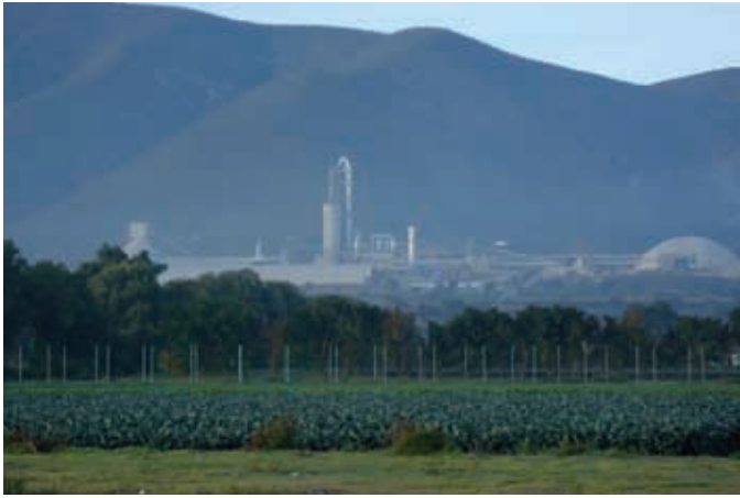
The new Cementos Cruz Azul plant at Palmar del Bravo, Puebla, Mexico, will produce 3,000 tons of cement per day when in full production.
