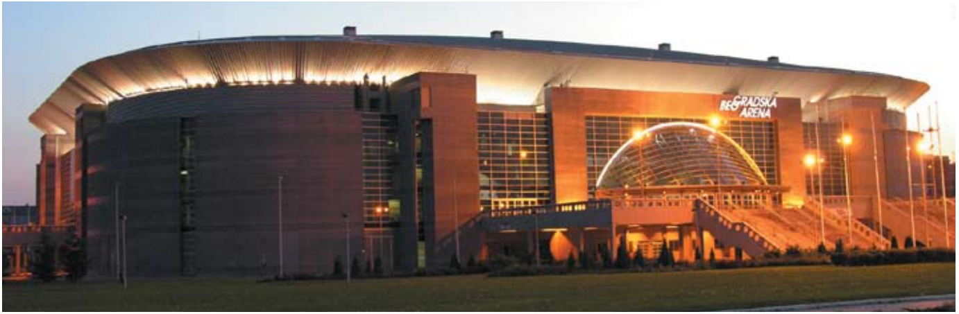
Four 500 kVA generator sets, organized into two pairs, each cover the power needs for half the arena.
