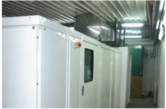
The generators housed in the basement feature soundproof enclosures to limit noise levels.
