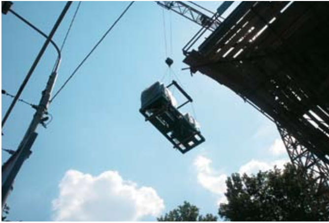
Special steps were taken to maneuver the large genset into the theater's basement.
