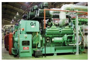
The generators were installed as a turn-key project by Cummins Power Generation that included the complete electrical and mechanical installation.
