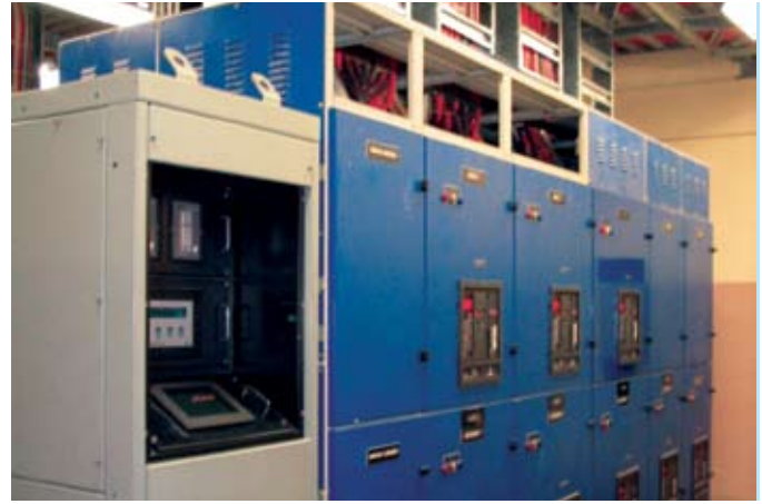
The PowerCommand Digital Master Control MC 200 synchronizes the operation of the gensets.
