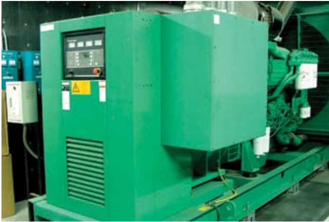
Cummins Power Generation gensets provide emergency backup to My Dinh National Stadium.
