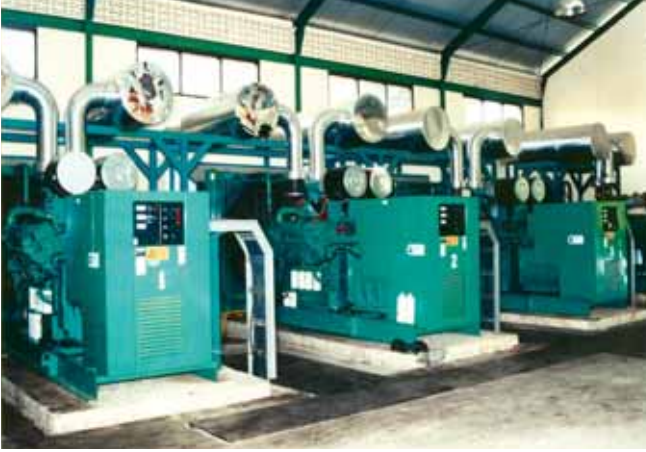
Cummins Power Generation high capacity gensets supplement power to the PLN supply at Bontang.
