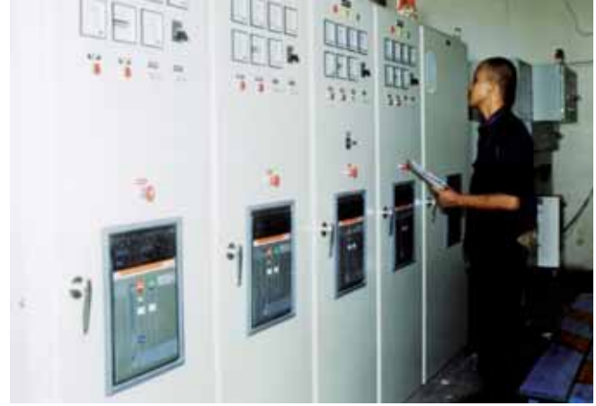
Paralleling switchgear facilitates synchronisation of gensets with the grid supply.
