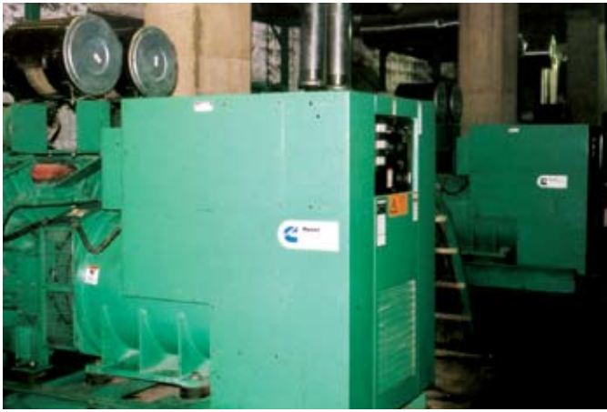
Five Cummins Power Generation gensets are operated daily to provide power for the mall.
