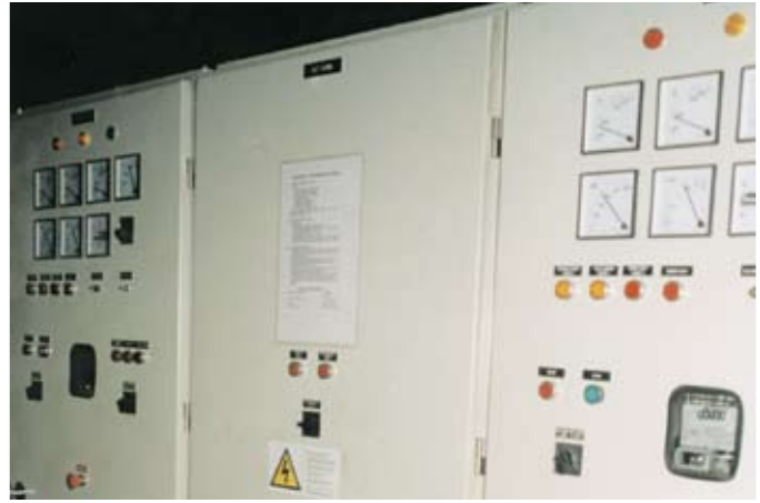
Paralleling switchgear ensure optimal use of gensets based on load requirements.
