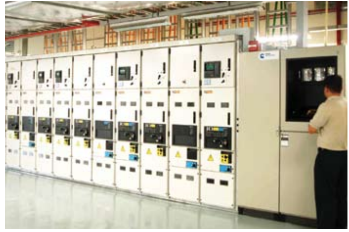
Cummins Power Generation advanced PowerCommand Control and ATS ensure load crossover within 20 seconds.
