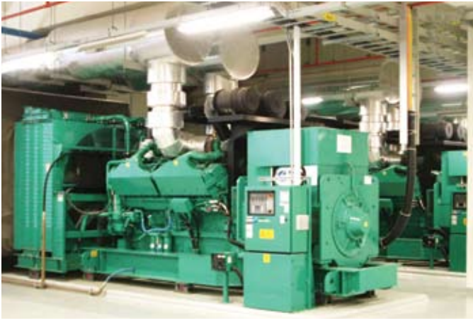
Cummins Power Generation high voltage generator system installed in UMCi.
