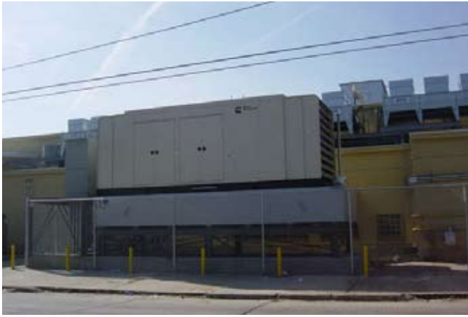
The generator is housed in a quiet, weatherproof container and sits atop an eight-foot-high, flood-protected platform.
