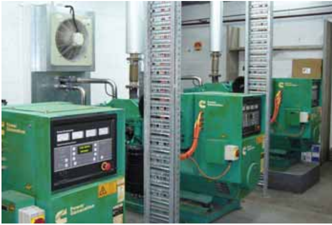
The fully integrated power system utilizes three Cummins Power Generation generator sets, Cummins PowerCommand digital paralleling equipment, and a Cummins digital master control system which is integrated in a new paralleling and distribution switchboard.
