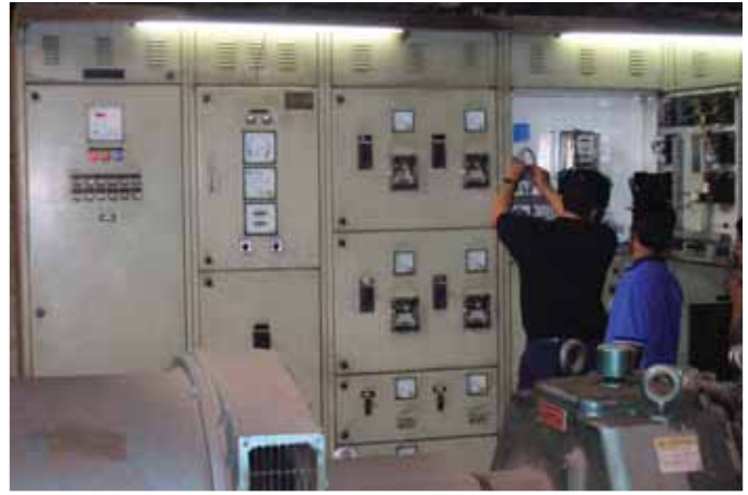
Technicians putting the finishing touches to the control wiring.
