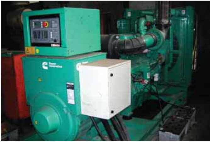
C550 D5 genset installed and ready for paralleling with the steam turbine.
