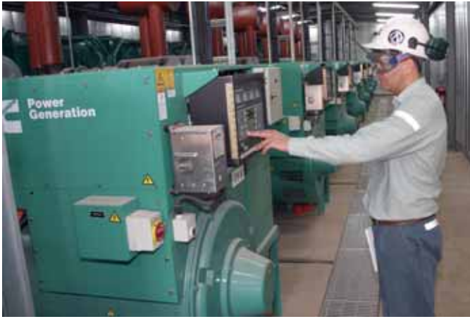
QAL senior project electrical engineer Craig Stevens interrogates the Cummins PowerCommand® genset control system.
