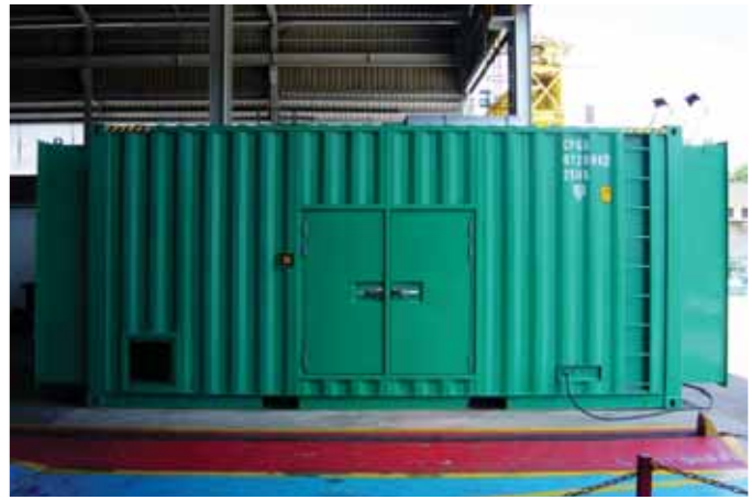
Cummins Power Generation C1500 D6 gensets powered by KTA50-G9 engines.
