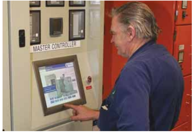
Cummins Power Generation DMC 200 provides plant operators with a touch-screen interface to monitor the gensets as well as system load and status.
