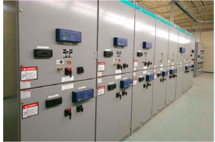
The system employs a switchgear pair that parallels the generator sets and connects them to the 27 kV step-up transformer for distribution.
