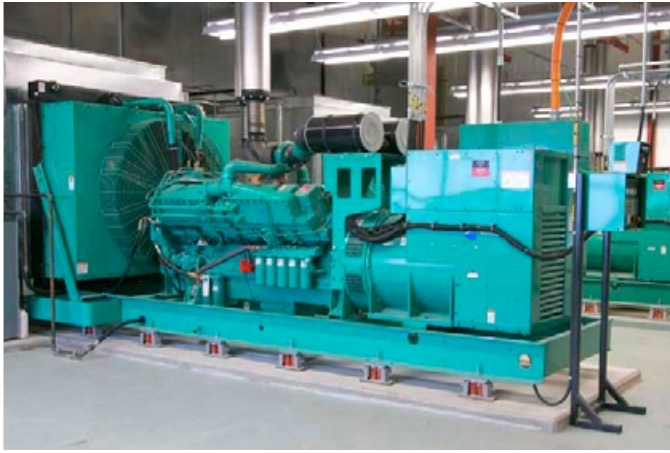
The standby power system consists of three 1250 kW Cummins Power Generation generators producing a total of 3.75 MW.
