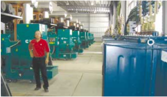
Installation of nine C2000 D6 generator sets
