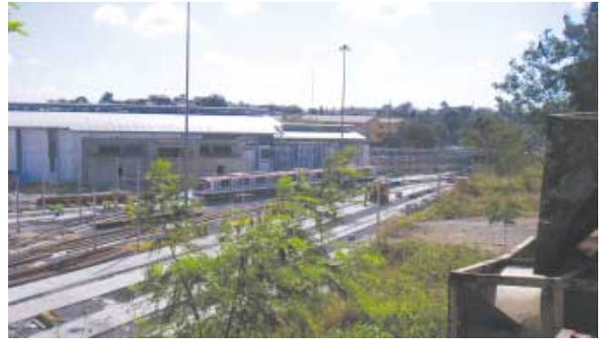
The C2000 D6 generator sets provide 18 MW of standby power to the entire Metro system
