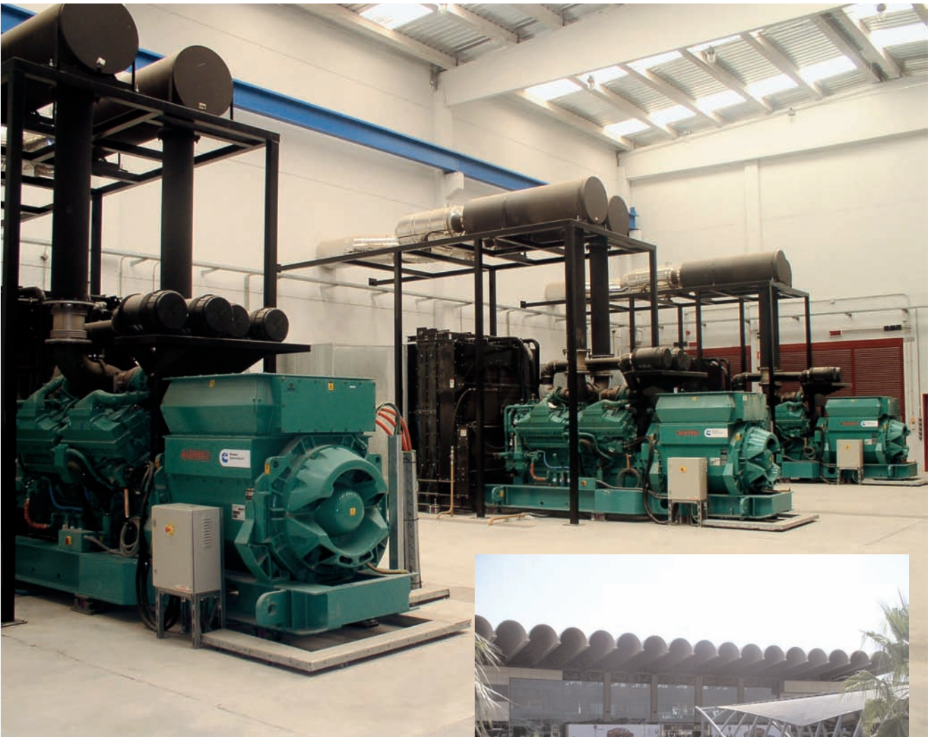
C2500D5A generator sets provide 6 MW of emergency standby power
