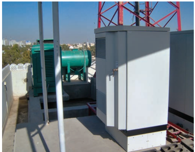
Installation of C33 D5 generator set
