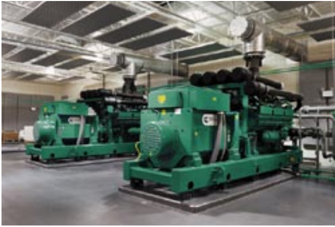
Michigan water plant keeps taps flowing and lowers costs with 5.4 MW standby power system from Cummins Power Generation
