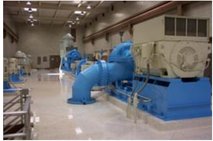
In an outage, these pumps are restarted after a 10-minute delay, while water storage tanks throughout the distribution system prevent any noticeable decrease in water flow to consumers.
