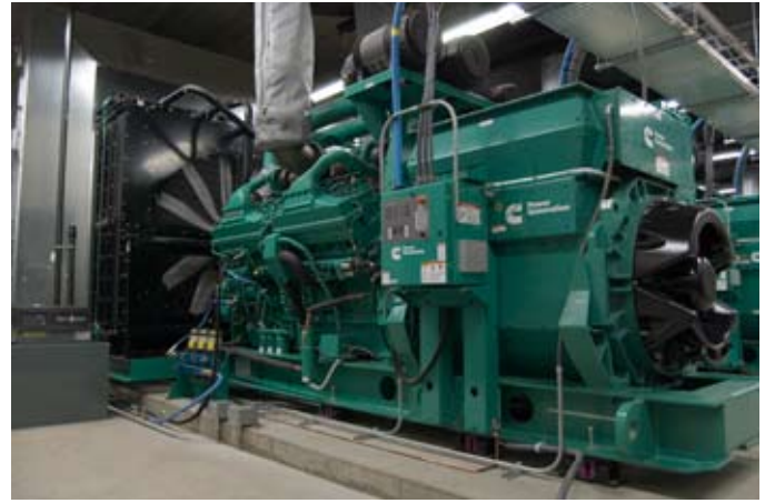
A 7,500-square-foot building houses the nine generators that can support a total load of 18 MW.
