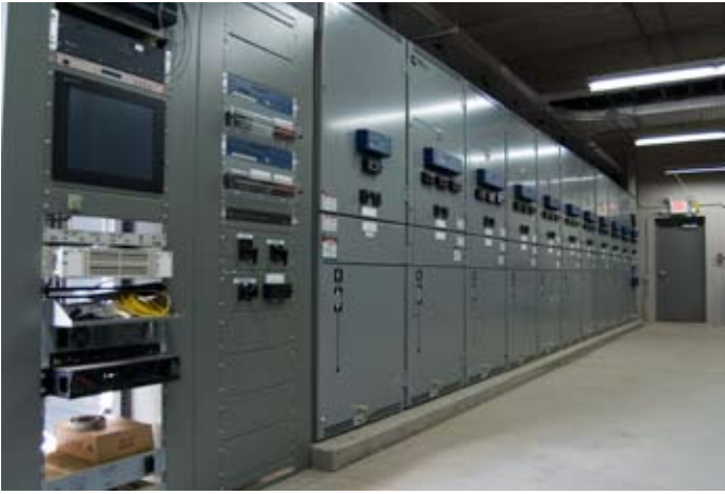
The switchgear at the Arrowhead facility allows the site to be reliably and remotely monitored and controlled from GRE's system control center five hours away in Elk River, Minn.
