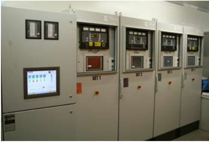
A Cummins Power Generation DMC300 Digital Master Control system is used for load demand management of the complete power station.
