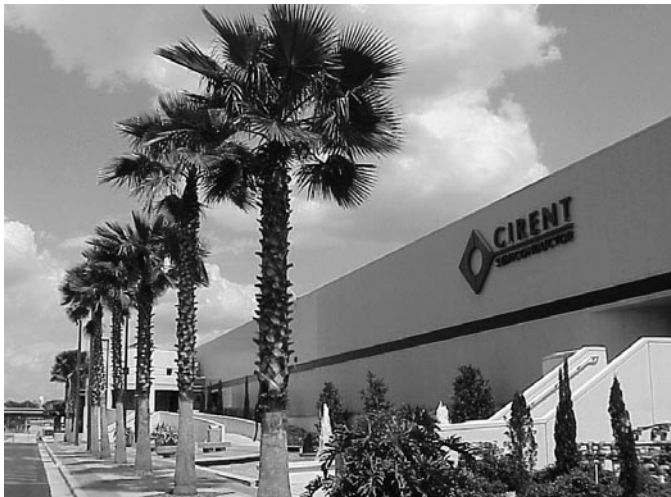
Cirent Semiconductor in Orlando, FL, has a 6 MW standby power system to prevent costly raw material losses during a utility outage.
