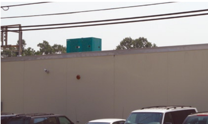
Rooftop installations, when possible, represent one solution to elevating a standby generator above flood waters in low-lying areas.
