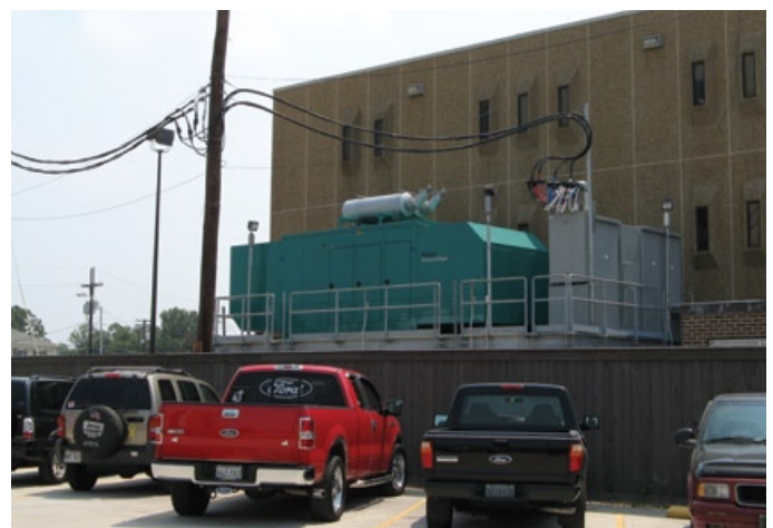
This platform installation takes advantage of a unique space created by a retaining wall in an urban area.
