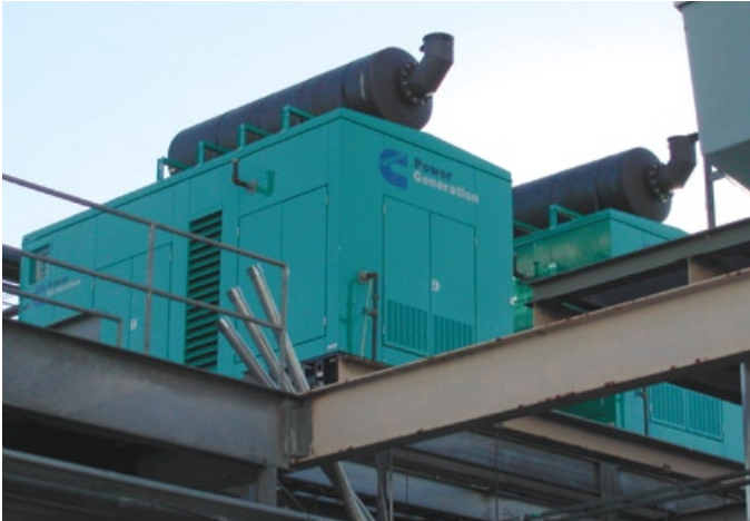
These generators are located on a high superstructure in an area where flooding is likely during severe weather.
