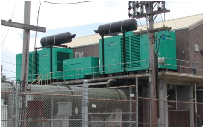
Three Cummins Power Generation generators at a Jefferson Parish canal pumping station were located above the maximum high-water level and continued to operate as long as they had fuel.
