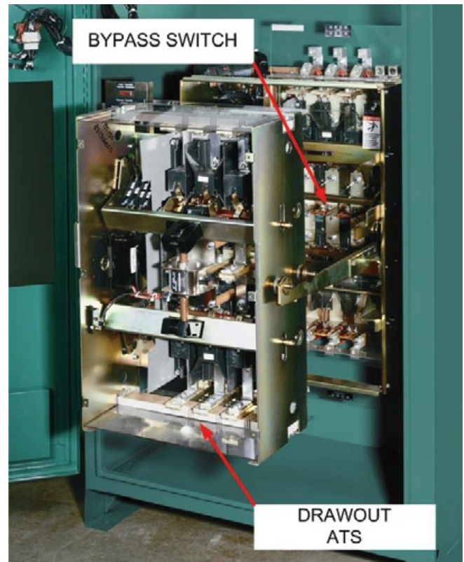
Figure 5 - Bypass/isolation transfer switch
