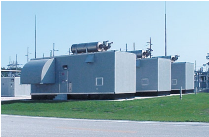
A semiconductor manufacturing facility in southern Florida relies on painted aluminum enclosures to provide corrosion-resistant weather protection.
