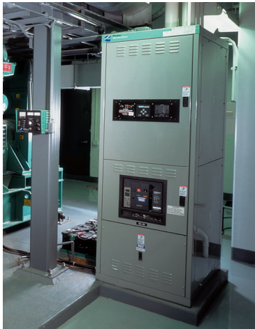
FIGURE 3 – Switchgear required for single generator set utility paralleling operation – peak shaving.
