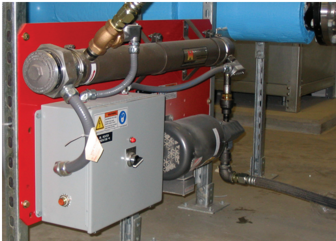
FIGURE 2 – Optional oil heater may be required to maintain the sump oil temperature at a level to facilitate quick start and run up.
