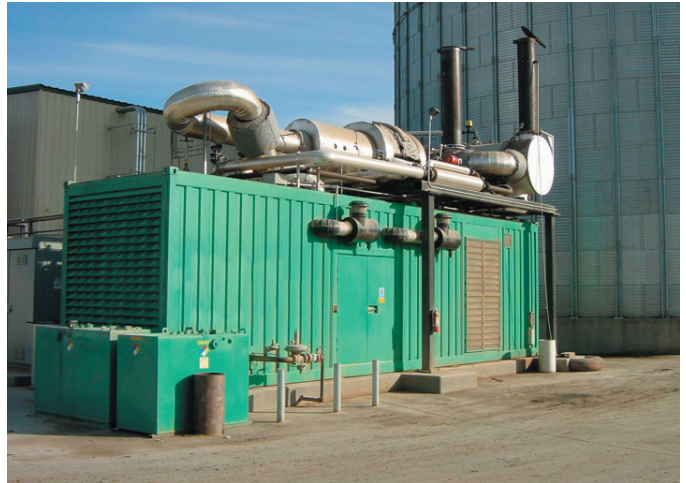
FIGURE 4 – Custom packaged LBNG CHP system.
