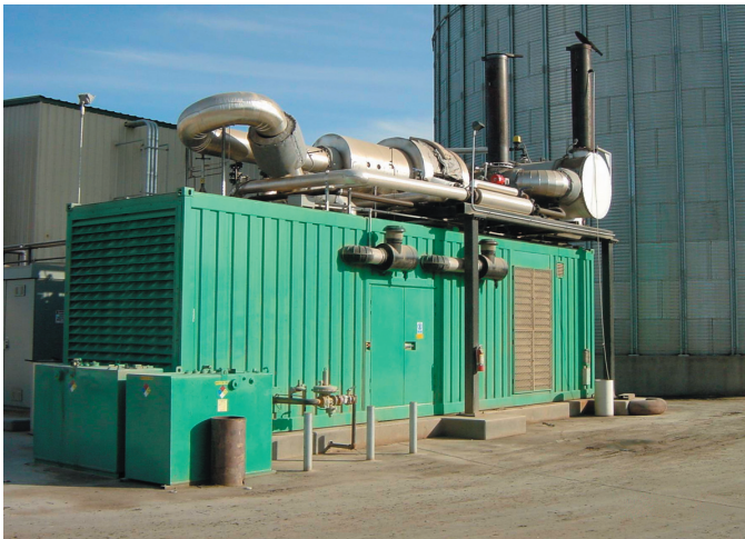
FIGURE 1 – Custom packaged lean burn natural gas CHP system.
